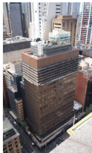
Upgrades begin at 20 Martin Place. Photo: Built
